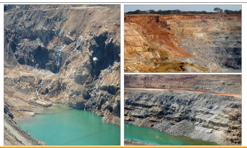
Poor pit condition with unstable, steep gradient. A number of pit failures have occurred.
